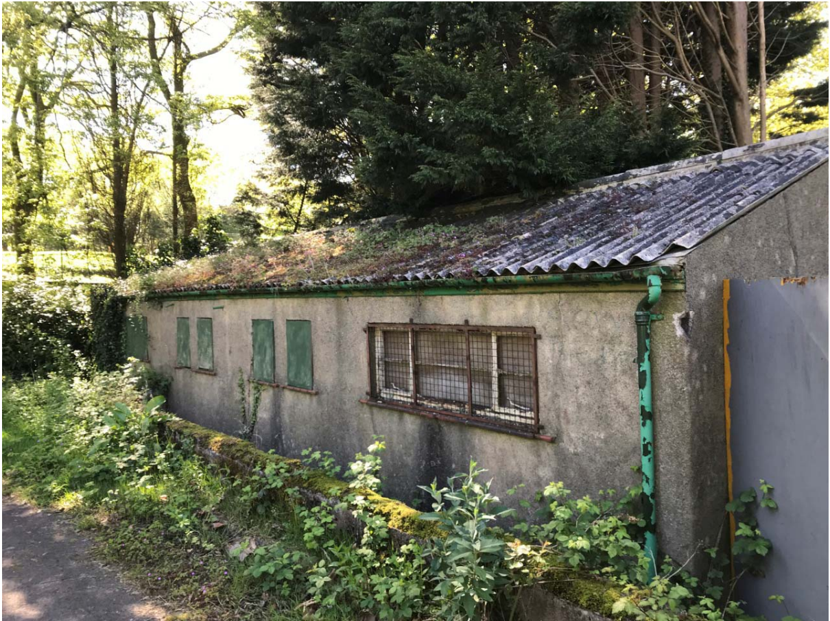
Remaining redundant building
